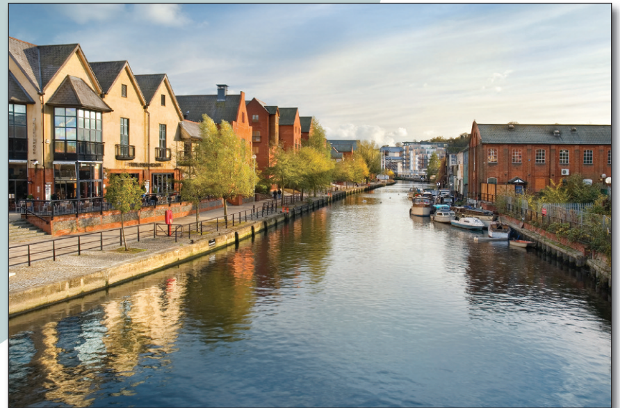
The view from Lady Julian Bridge, looking towards the Novi Sad Friendship Bridge.
